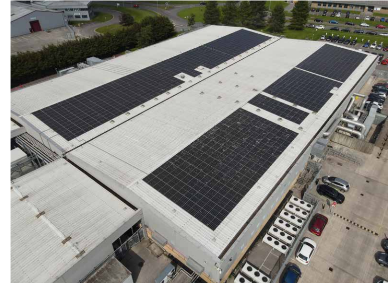
Waterton office solar panel — UK
